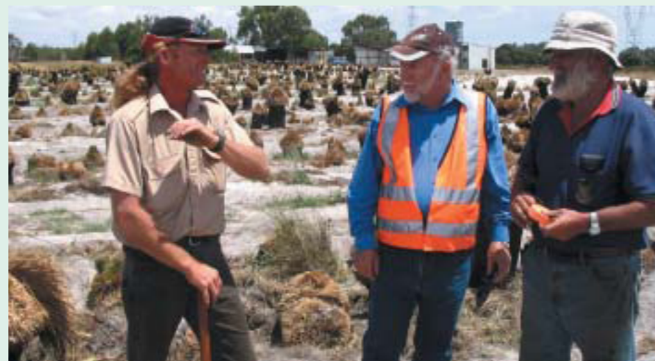
Excavator operator Ray Poole, Contracts Coordinator Bevan Curley and Supervisor Boots Kilroy with the grass trees saved for rail landscaping
