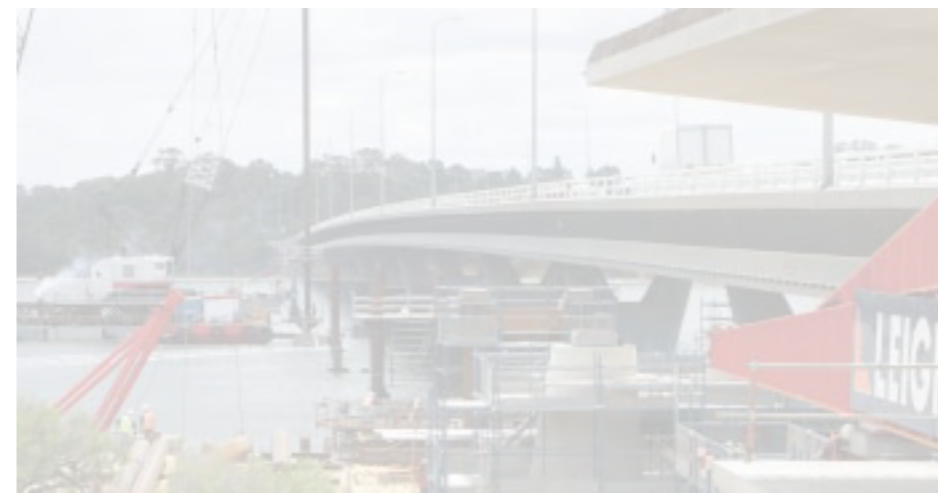
The Mount Henry Bridge works
